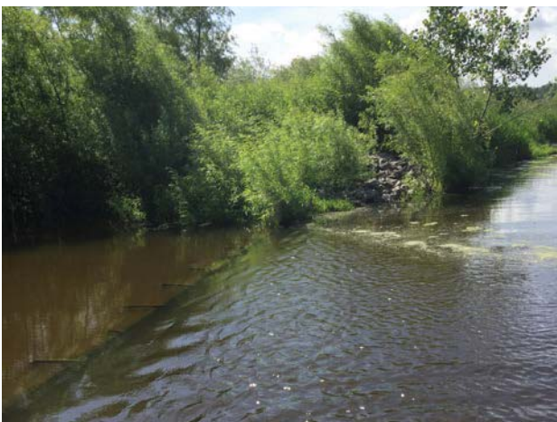
Existing water control structure.
